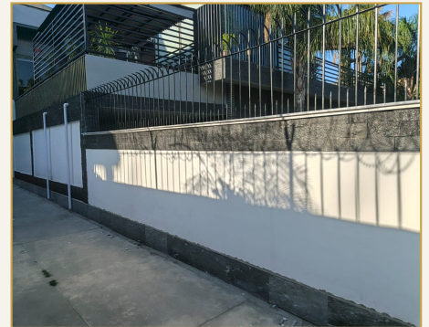
Boundary wall with steel railing
