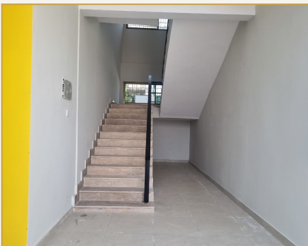
Interior staircase & landing
