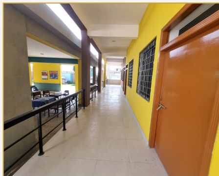
Finished corridor with door work
