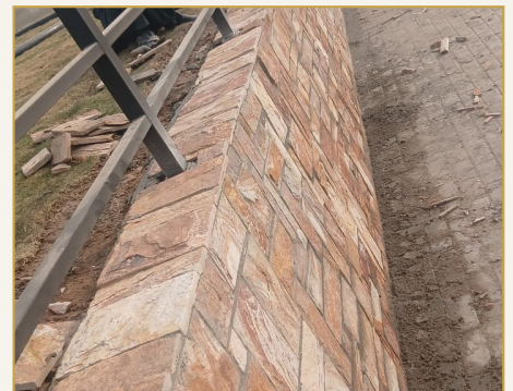
Natural stone boundary cladding
